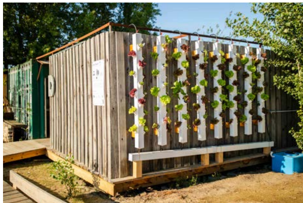
This blue-green prototype in the Park am Gleisdreieck uses greywater for the vertical cultivation of lettuce.
