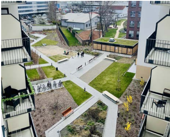
System setup of retention green roof in the backyard on top of an underground parking garage, which can store large amounts of water in case of heavy rainfall and thus provide needed irrigation water.
