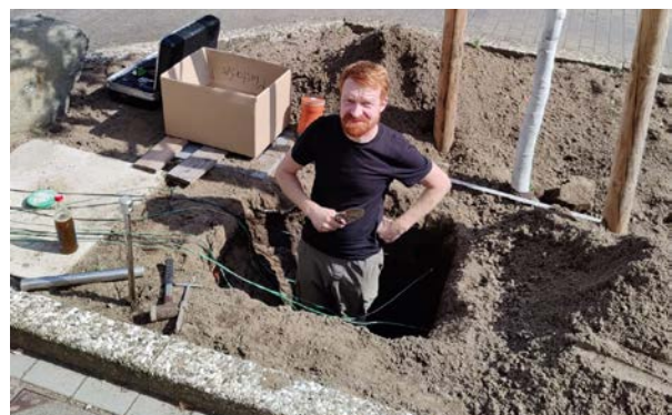
Installation of sensors for soil water balance measurement in a pilot tree pit.
