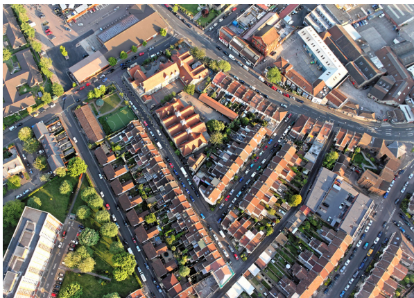
Resource-efficient urban districts – proposed solutions for water management, area and material flow management
