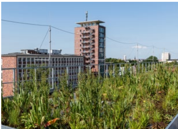
Green roof - example of multifunctional blue-green infrastructure: Energy supply, water retention, water storage, evaporation
